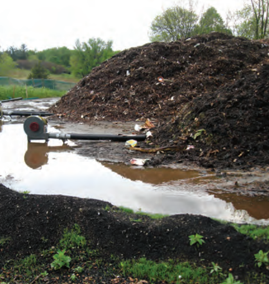
A compost berm (far left) was installed to measure how effective the berm was for treating contact water.
