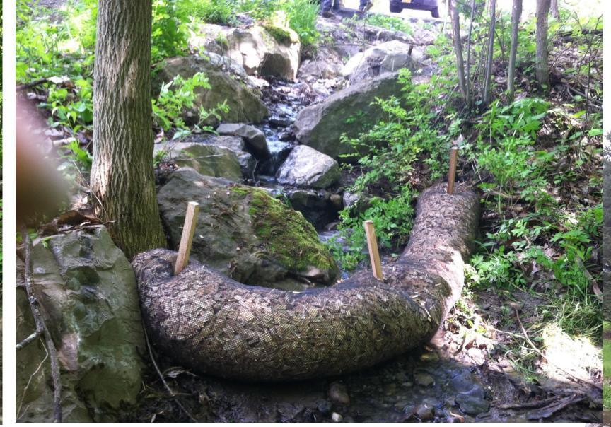
Organic matter in "socks" along waterways prevents erosion of banks and keeps contaminants out of surface water.
