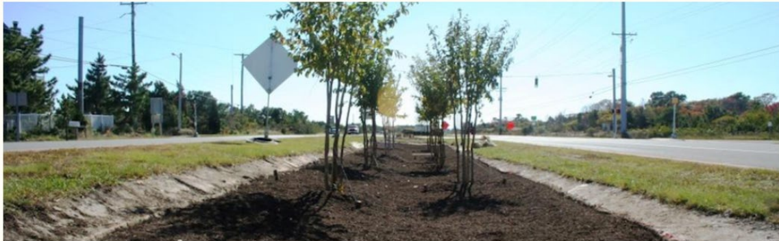
Storm water retrofits prevent water from washing into storm drains, allowing it to soak and filter into the ground.
